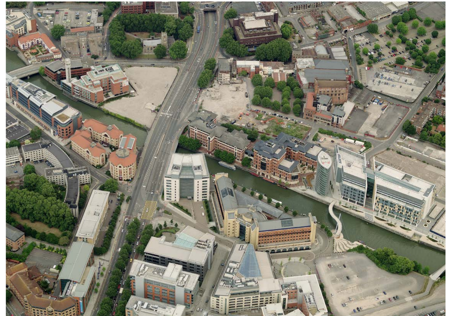
Fig 14: Temple Quay -existing aerial photograph from the south
