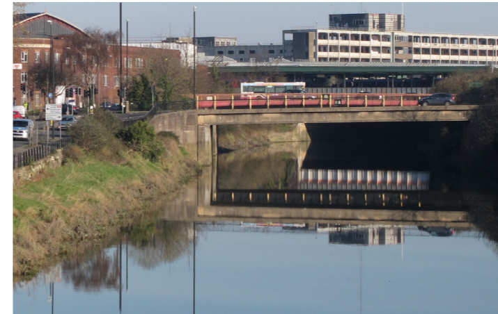
Flood risk, predominantly the tidal influence of the River Avon and New Cut
