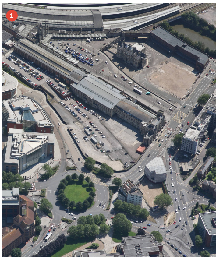
1 Temple Circus, Plot 6 and Station Approach present significant opportunities for public realm enhancement
